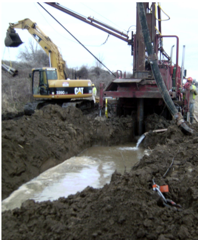
Discharge pit and drill rig in action at above Cairo relief wells.
